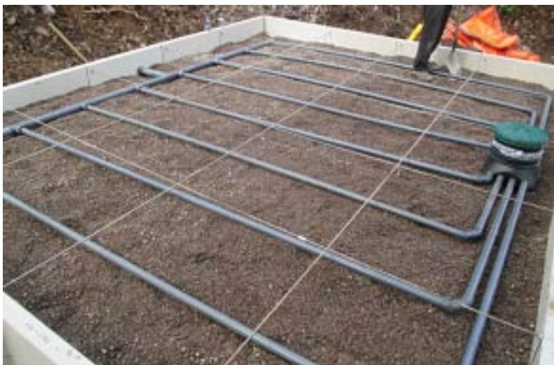
Fig 4.0 Completed pipe network on a Sandcel before placement of final gravel layer
