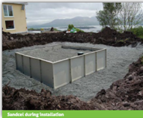
Sandcel during Installation
